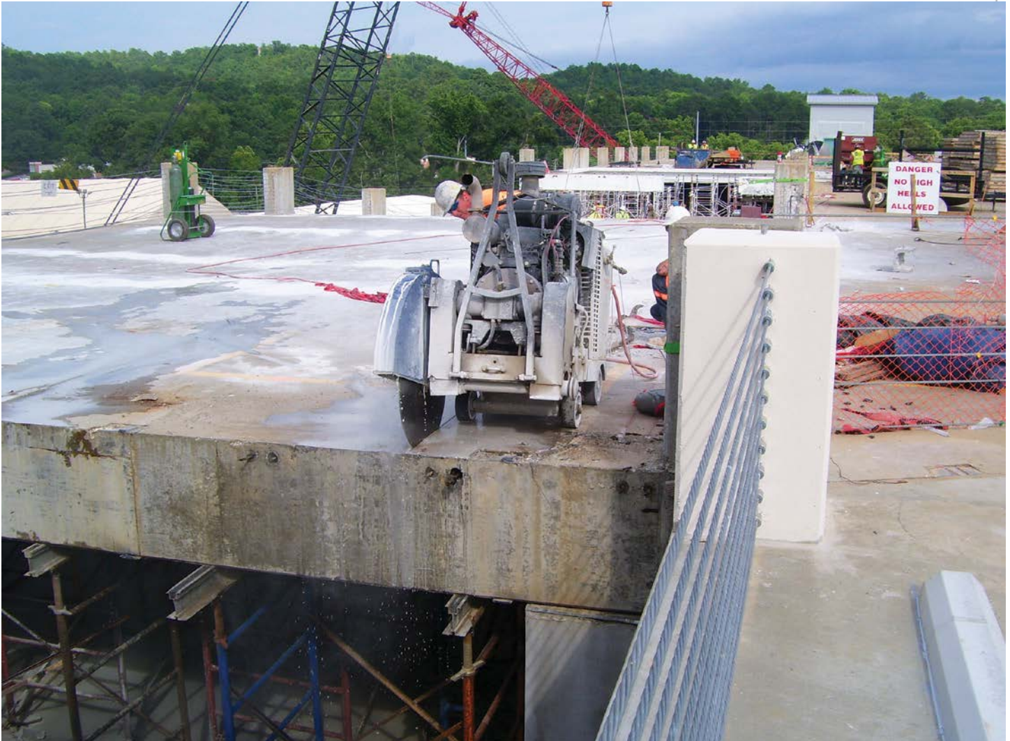
Slab decks were cut into 20-foot by 6-foot sections.
