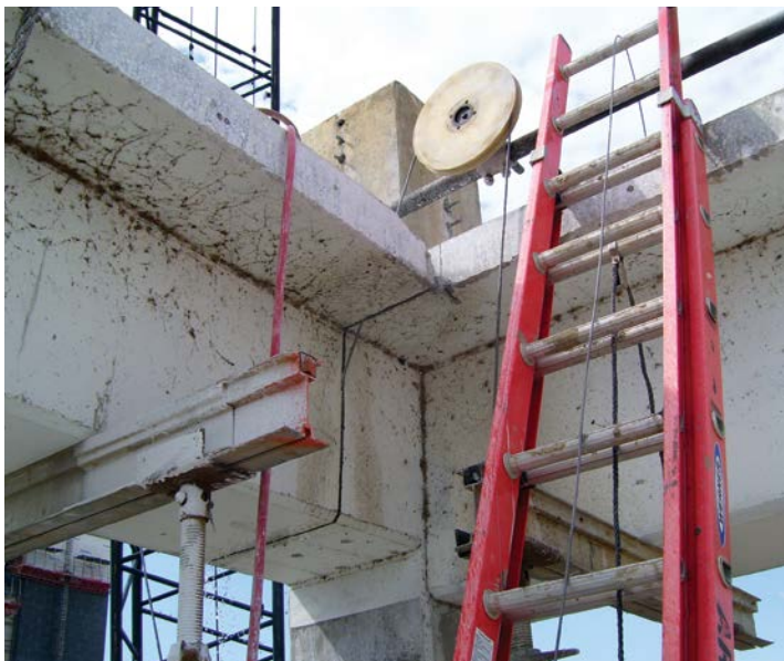
Wire saws were used to cut through support piers and beams.
