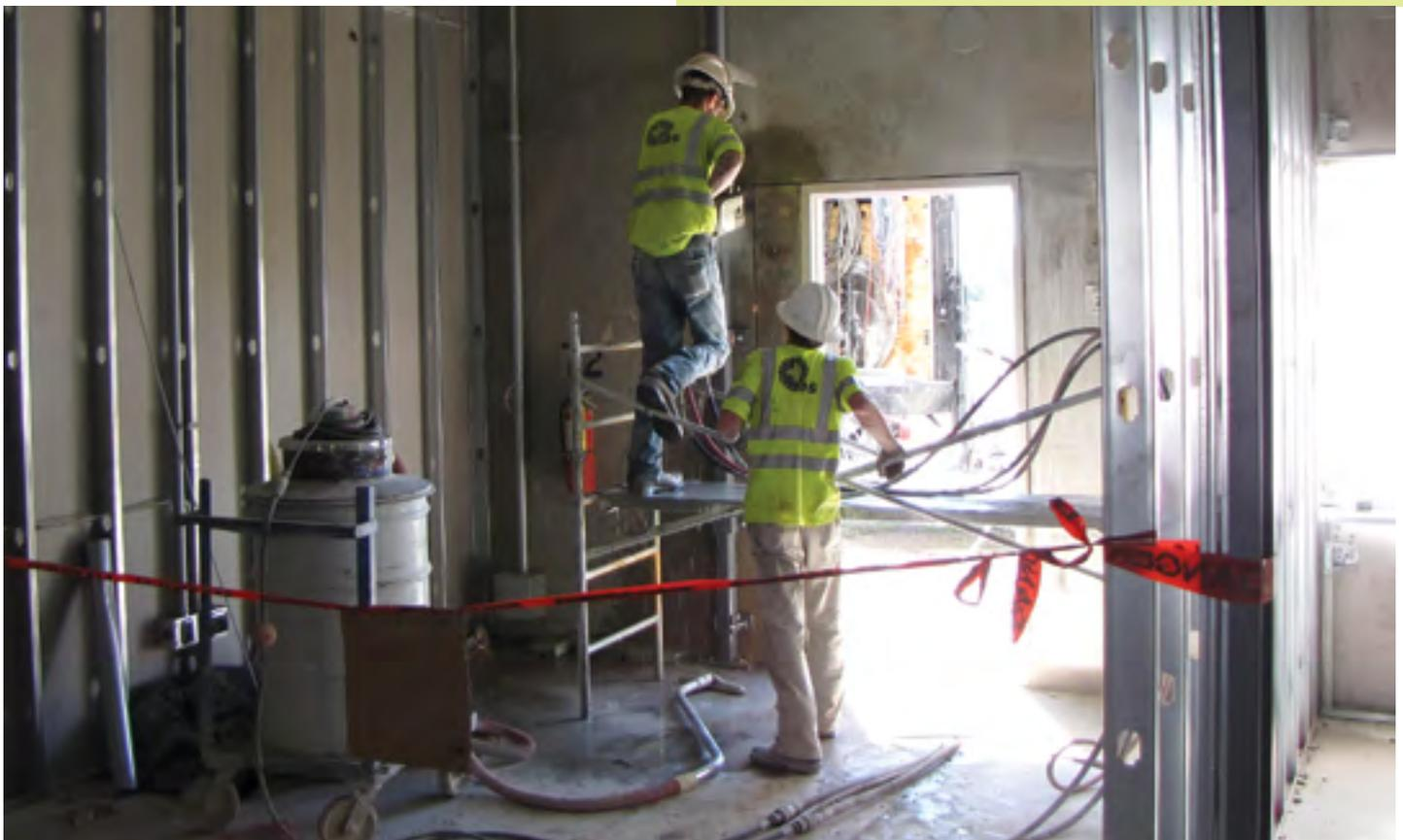
Operators employed concrete chain saws to make corner cuts in the openings.
