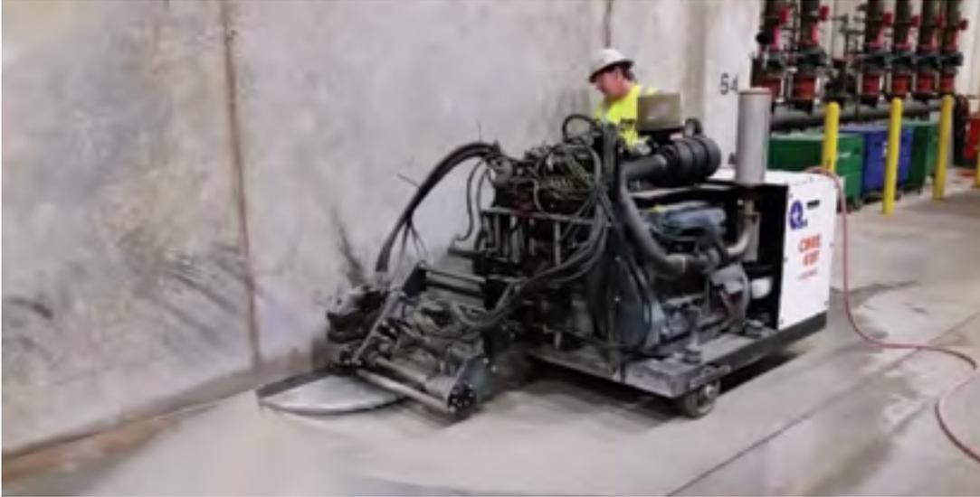
Dock door openings, some 14 feet square, required cutting flush with the slab.
