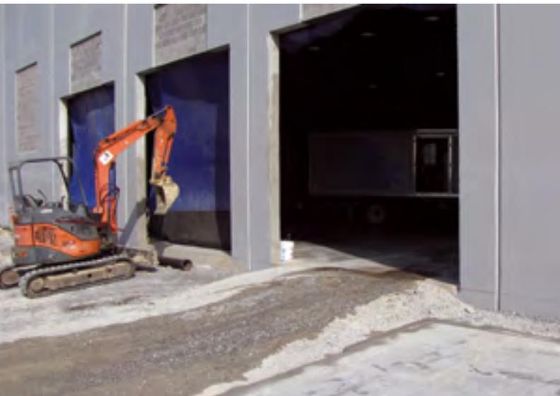
All window and dock door openings were made through 10-inch-thick precast concrete walls.
