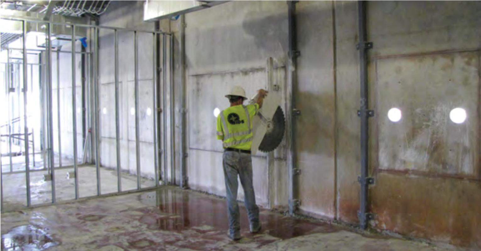
Track-mounted wall saws were used to create 5-foot-tall, 4-foot-wide window openings.
